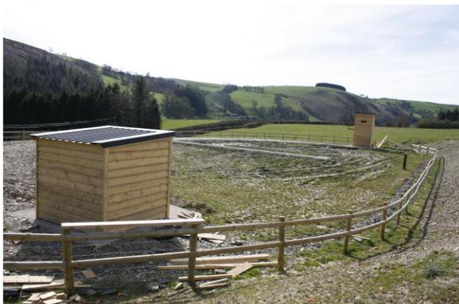
New Range – Olympic Skeet: The high and low towers are built and covered with featheredge boards cladded to the outside with corrugated galvanized steel roof to form weather proof building that blends in with the existing trap ranges and the natural environment.
